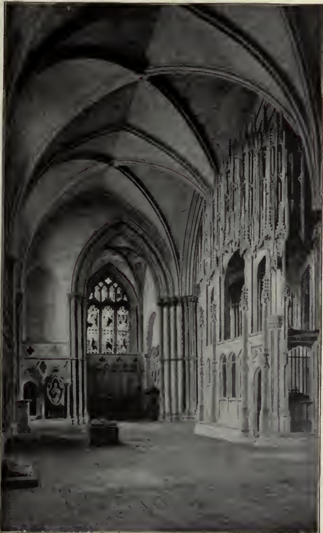
Photo, F. Frith & Co. Ltd. FIG. 15.—EARLY ENGLISH VAULTING. Winchester Cathedral, Waynfleet's Chantry. XXVII. 960.
